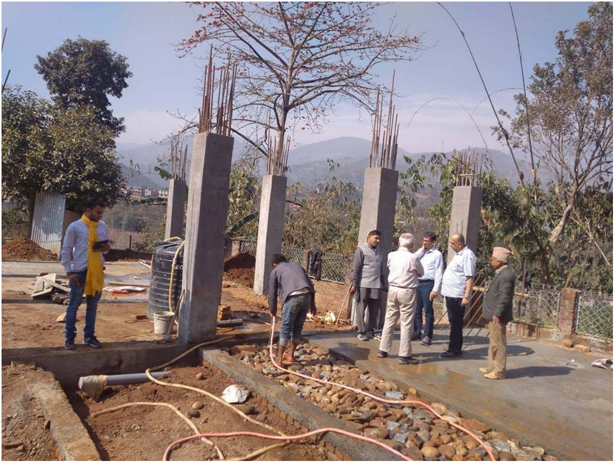
Sewa UK team at the construction site.
