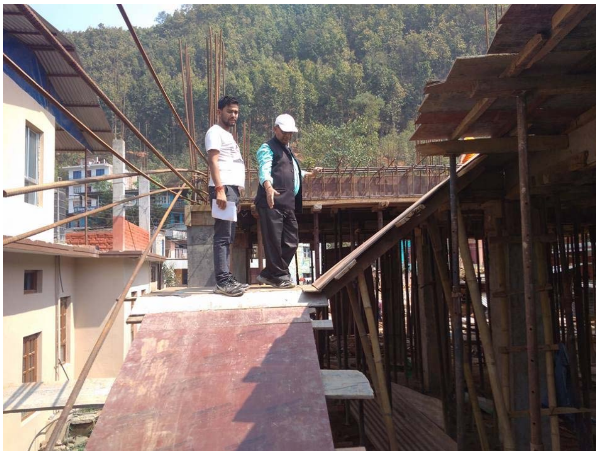
Engineer Shri Suresh Aggarwal (General Secretary, Sewa Nepal) at construction site.
