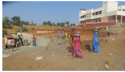
area where the residential building will be
