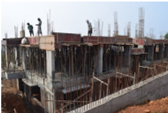
The work on the residential quarters
